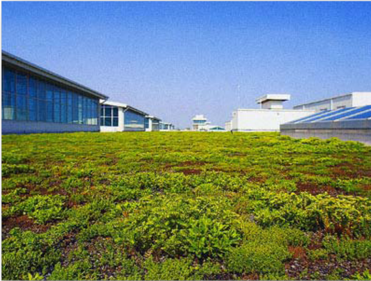
Extensive Green Roof
