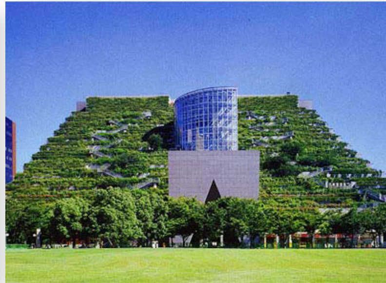
Intensive Green Roof
