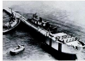
Flg floats normally while being towed into position by its flag. The tubular attraction is then filled with water to become a vertical support.
