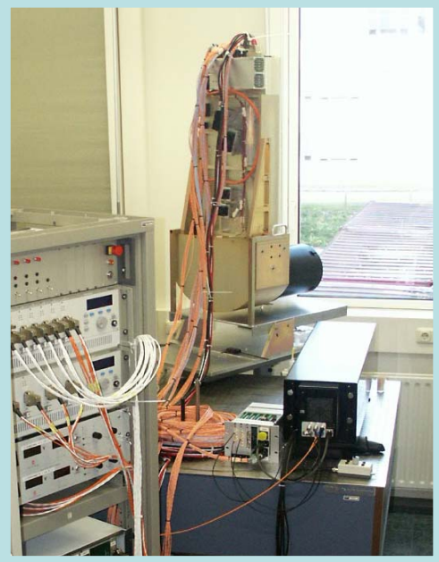
Data Recorder + RT Processing (FPGA)
