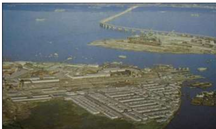
Fig. 2. Village for workers at the time of construction of the Rio-Niterói Bridge. Source: apud Freire, 2010
