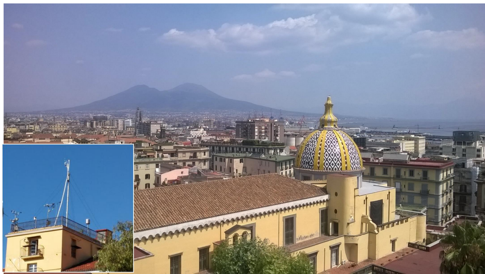
A view from the terrace where the instrumentation is setup. Bottom-left: the EC tower seen from an adjacent rooftop.
