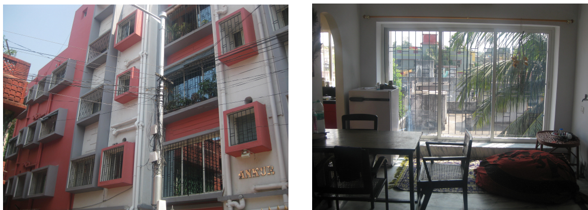
Figure 1a: Picture of the west facade. Figure 1b: Picture of the interior.
